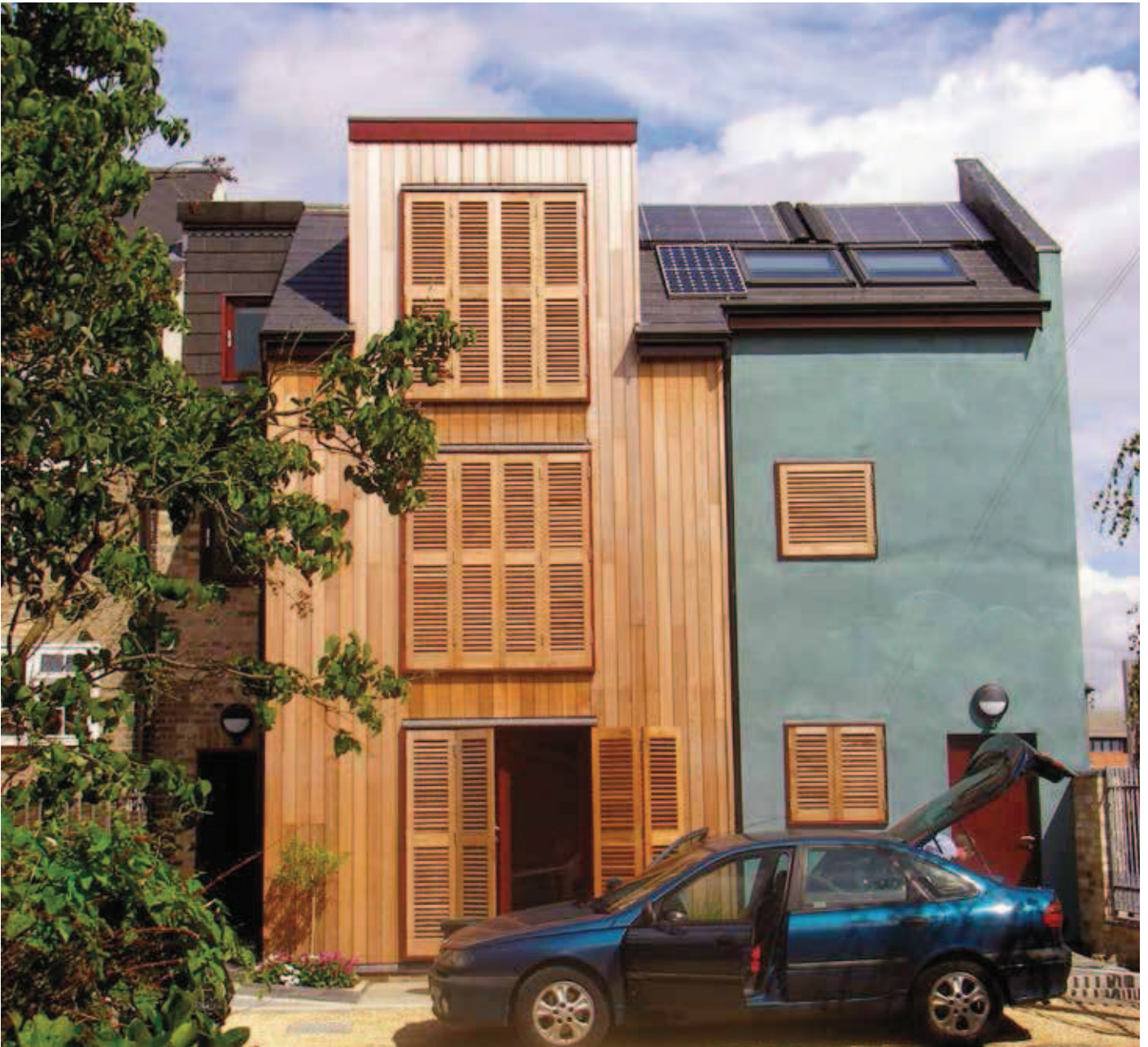
Figure 6 External shutters may become a necessary addition in the UK. Image courtesy of AC Architects.
